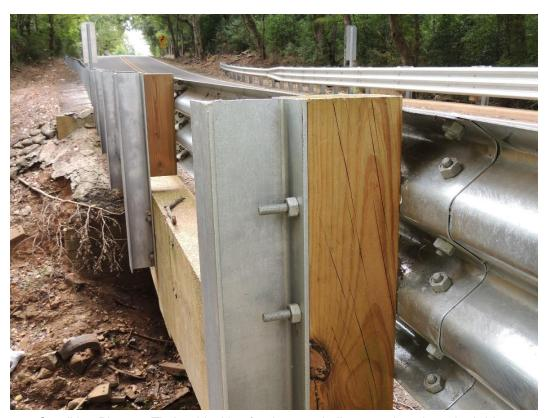
Condition Photo 9: Timber blocking for the guardrail connection along the bridge.
