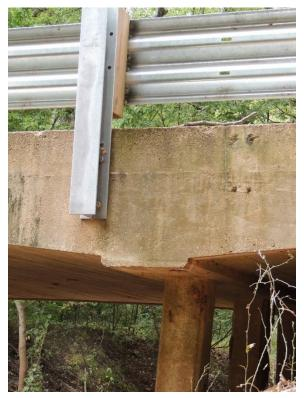
Character-defining Feature Photo 2: Close-up view of integrated pier cap poured monolithically with the concrete slab.
