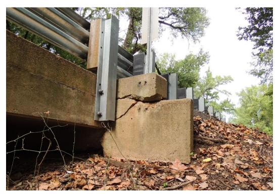
Condition Photo 4: Bent 4, east wingwall cracked and spalled with exposed steel, looking north.
